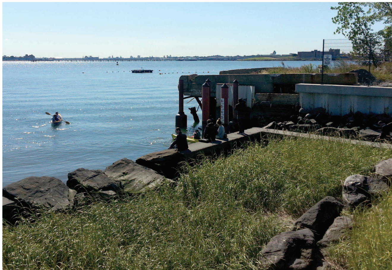
The constructed soft edge of Hunts Point Landing buffers development in the South Bronx from the East River while still allowing public access.
